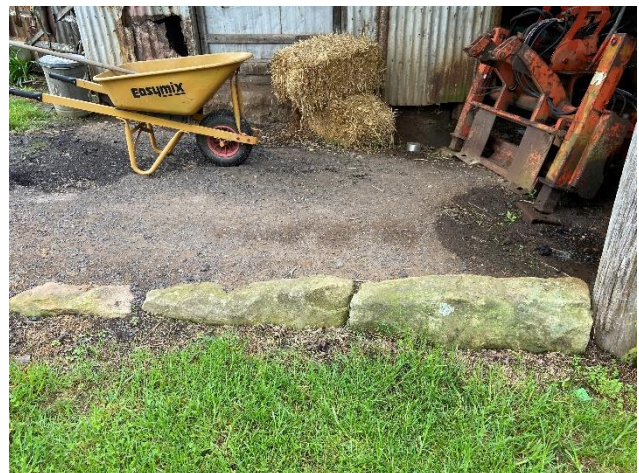
Plate 11: Original sandstone footings, facing north.
